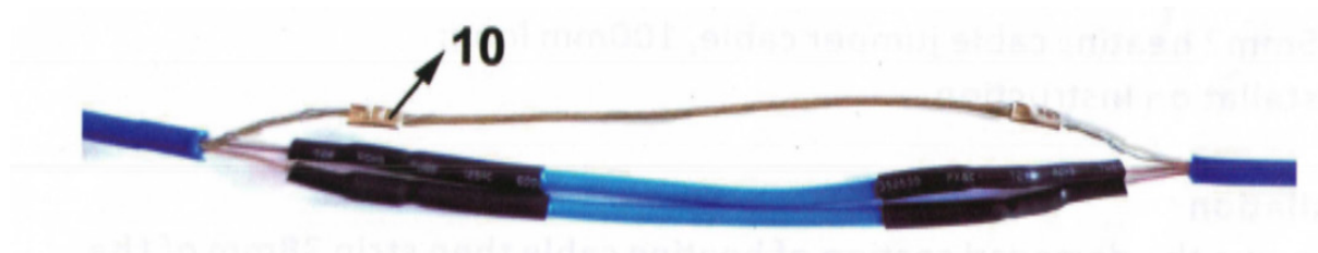
Step 10 - connection of the protective conductor/earth braid. Schematic illustration.
